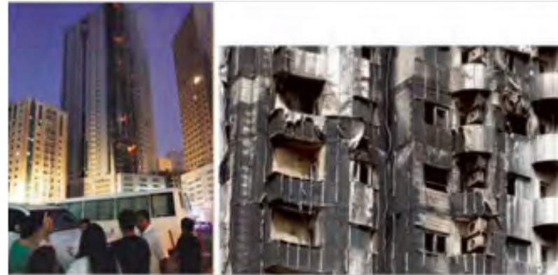
Fig. 5.13 Al Tayer Tower façade fire 2012 [49, 50]
