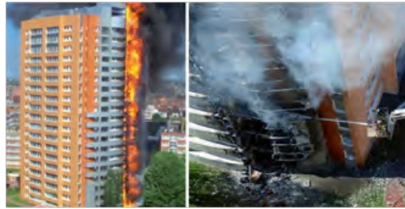
Fig. 5.12 Mermoz Tower during and after façade fire [45]
