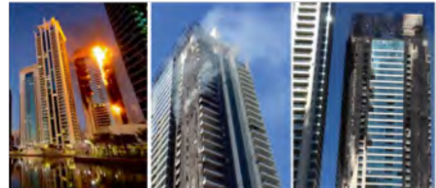
Fig. 5.16 Tamweel Tower fire 2012 [55]
